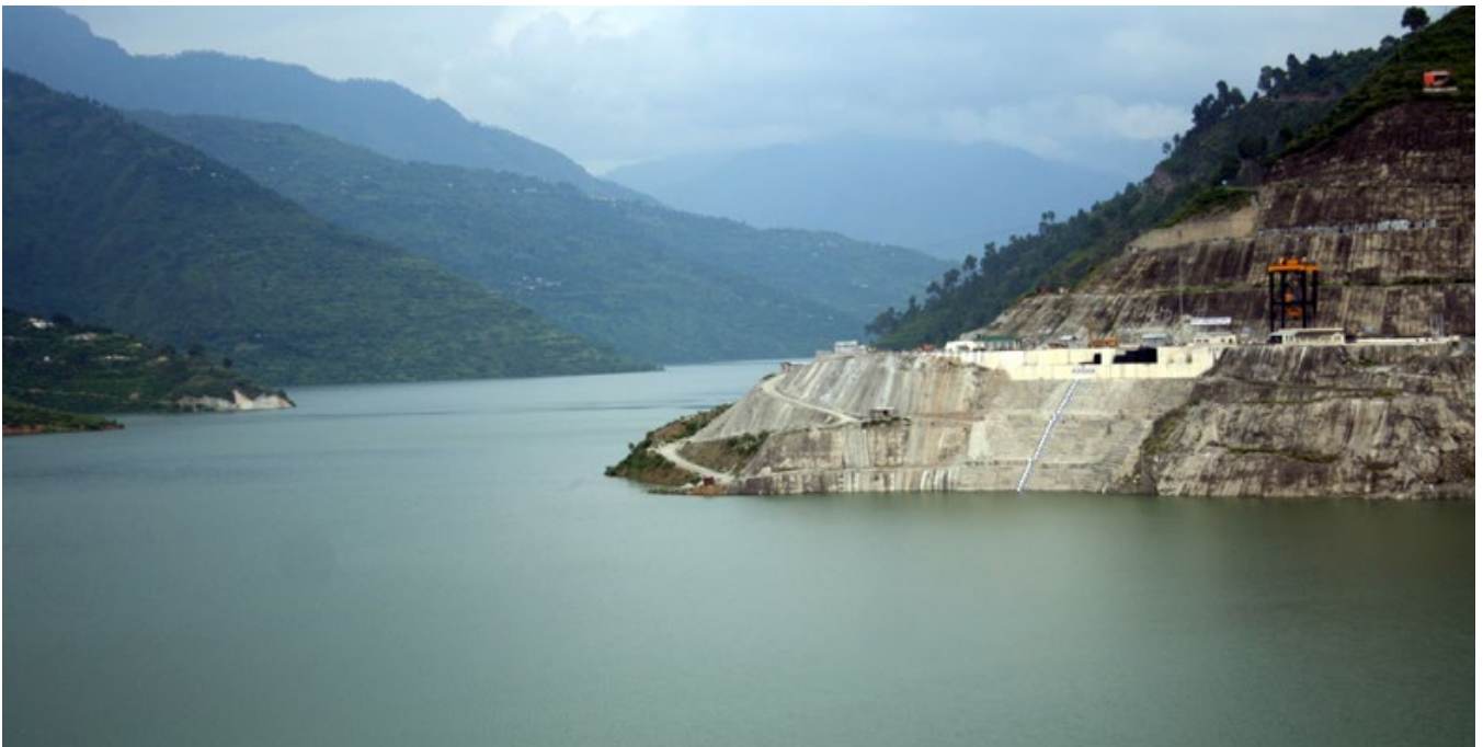
Image 5: Tehri Dam, Bhagirathi River, Uttarakhand. Source: Gaurav Arora–Tehri Dam, CC BY 2.0, https://commons.wikimedia.org/w/index.php?curid=4089090 .
